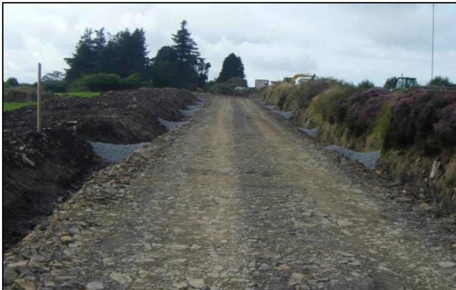
Plate 3-9: Example of a dirty water conveyance swale and check dam
