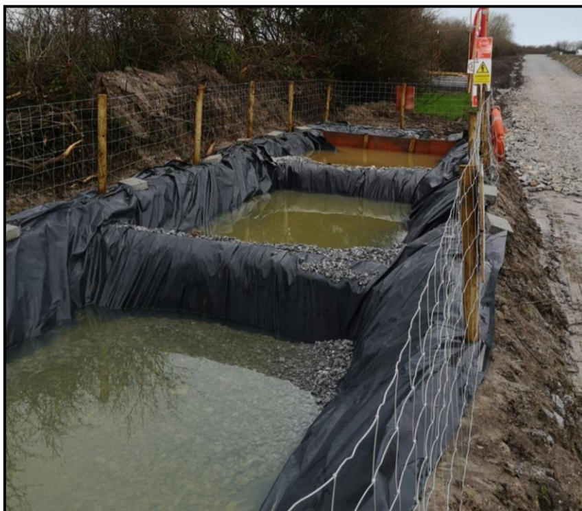
Plate 3-12: Example of a sediment settlement pond with stone filter
