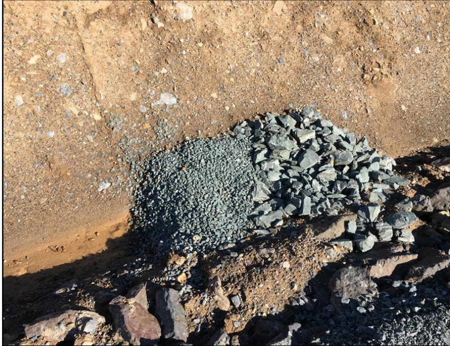
Plate 3-10: Example of a stone check dam with large aggregate on downstream side
