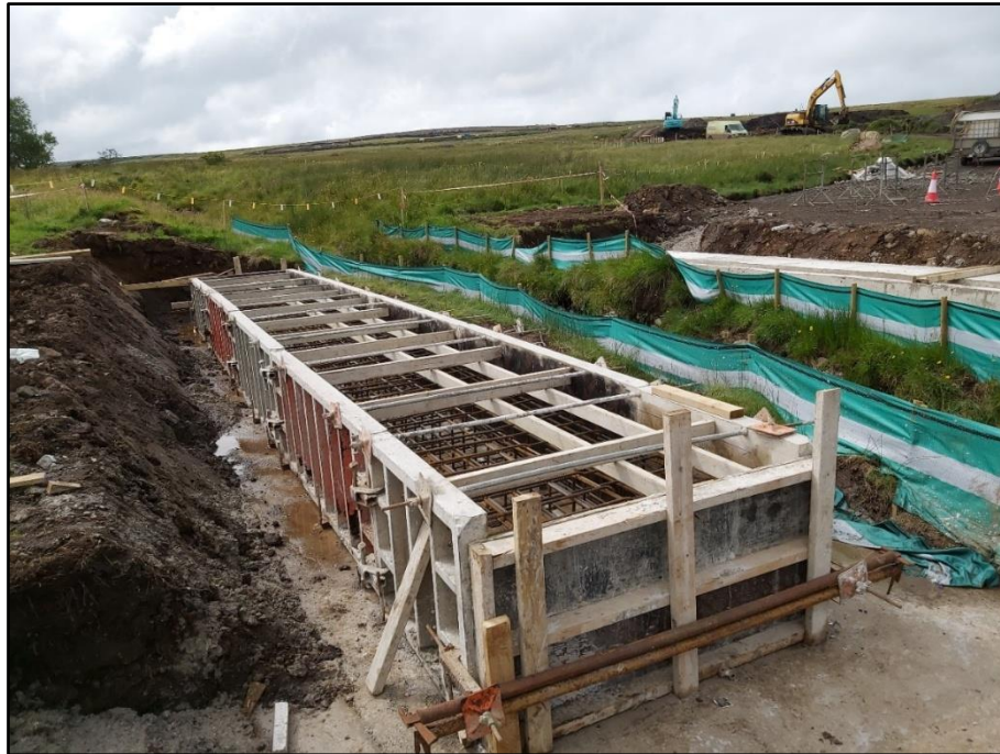
Plate 3-11: Example of a silt fence used on wind farms
