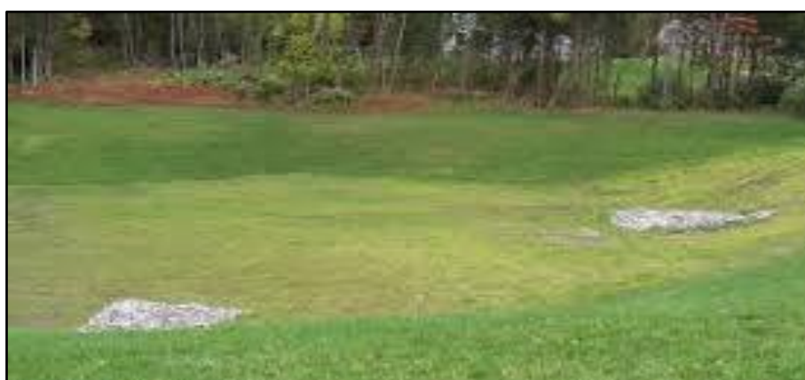
Plate 3-6: Example of a detention basin
