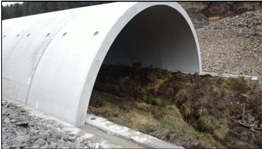
Plate 3-3: Example of a pre-cast concrete culvert in place over an existing watercourse
