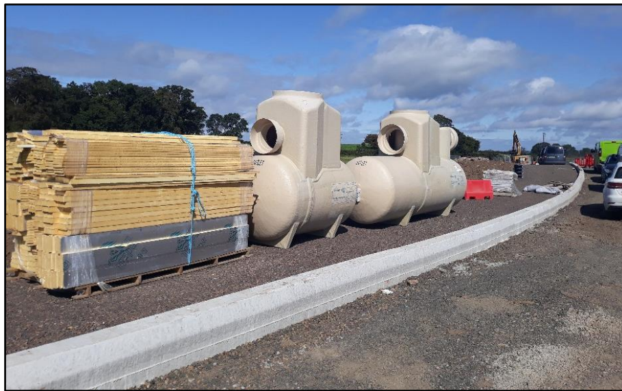
Plate 3-5: Example of a proprietary treatment device
