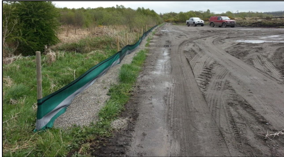
Plate 2-2: Example of a silt fence along existing tracks near watercourses
