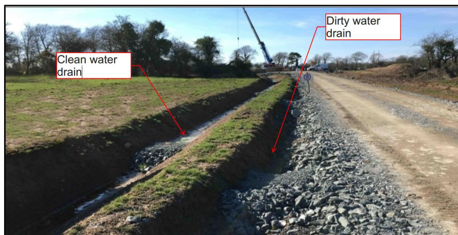
Plate 3-1: Example of wind farm clean and dirty water swale
